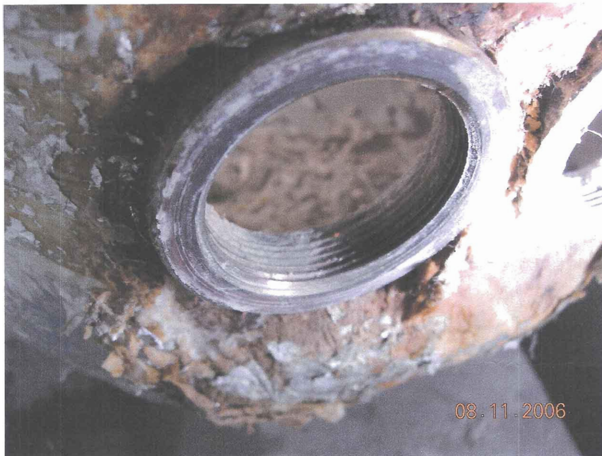
photo 1: The bottom of the steam drum
